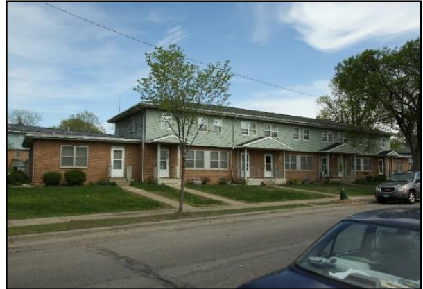
2821-2835 Delaware Avenue Southeast, Type F, view southeast.
