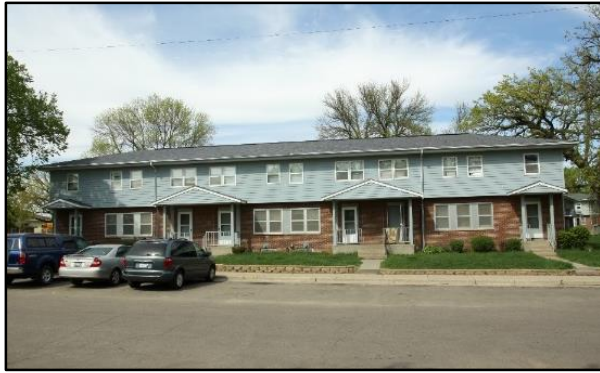
2801-2811 Saint Mary's Place, Type C, view northeast.
