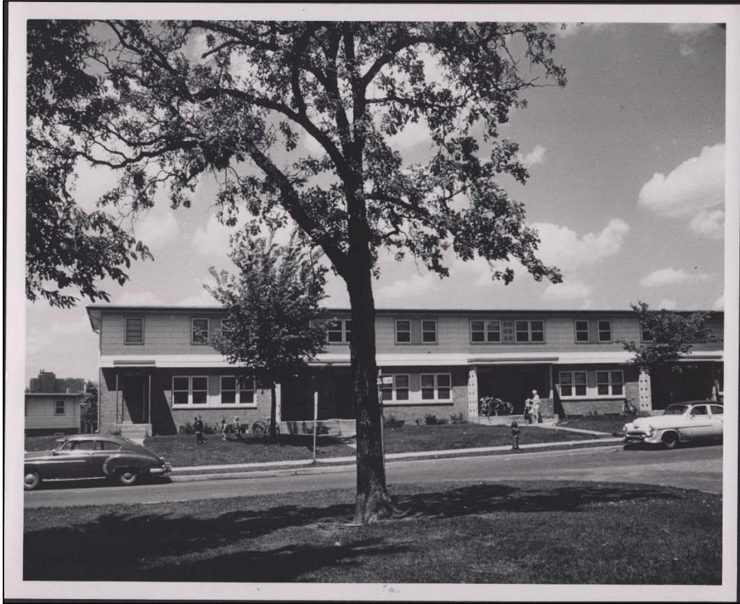
Unidentified townhomes at Glendale Public Housing, undated. (James K. Hosmer Special Collections, Hennepin County Central Library)
