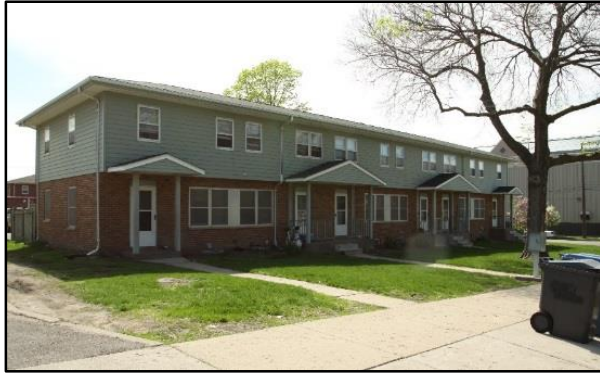
2700-2710 Delaware Street Southeast, Type A, view southwest
